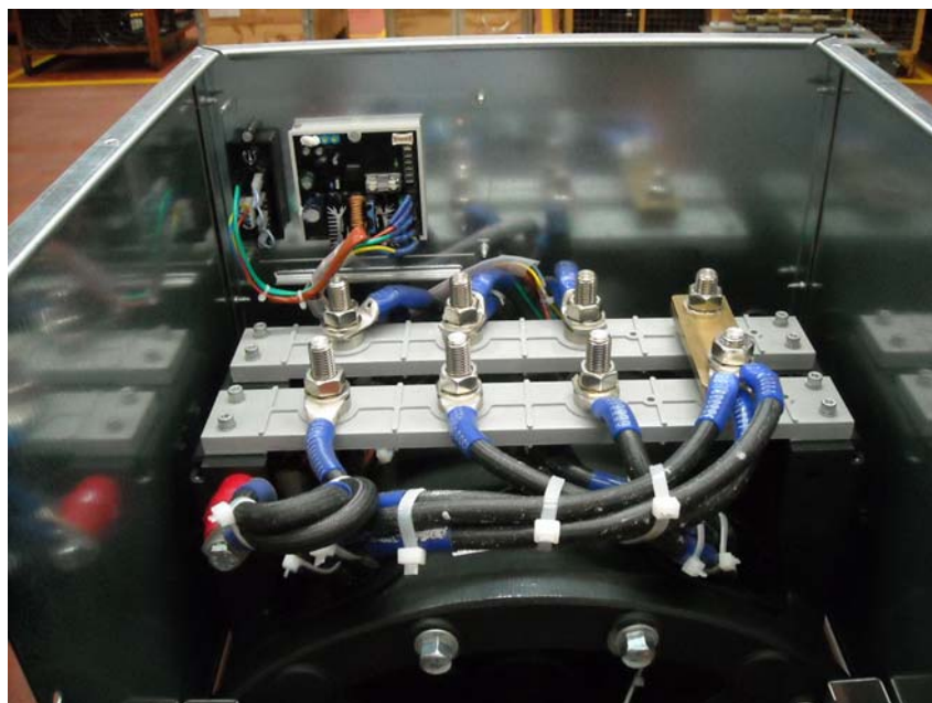
Fig.32 ECO38 lateral panels mounting detail
